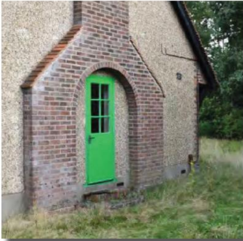
4.08: West chimney breasts gathering in round arch
